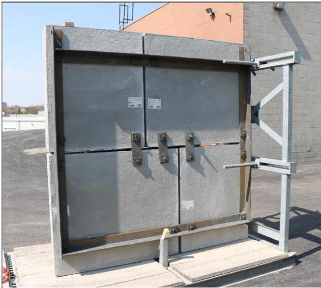
Figure 2.1 – Mock-up Wall 1, viewed from the indoor side, showing back of precast concrete panels and connections to steel frame.
