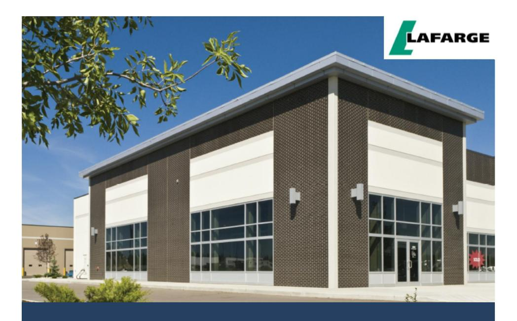
**INSULATED PRECAST CONCRETE WALL PANELS**
